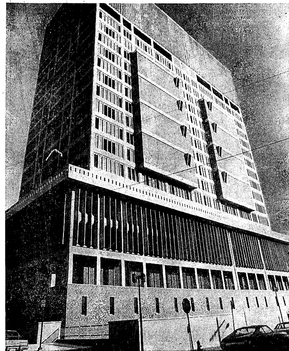
New Middlesex County Courthouse soars 22 stories into the air. (Globe photo by Jack O'Connell)
