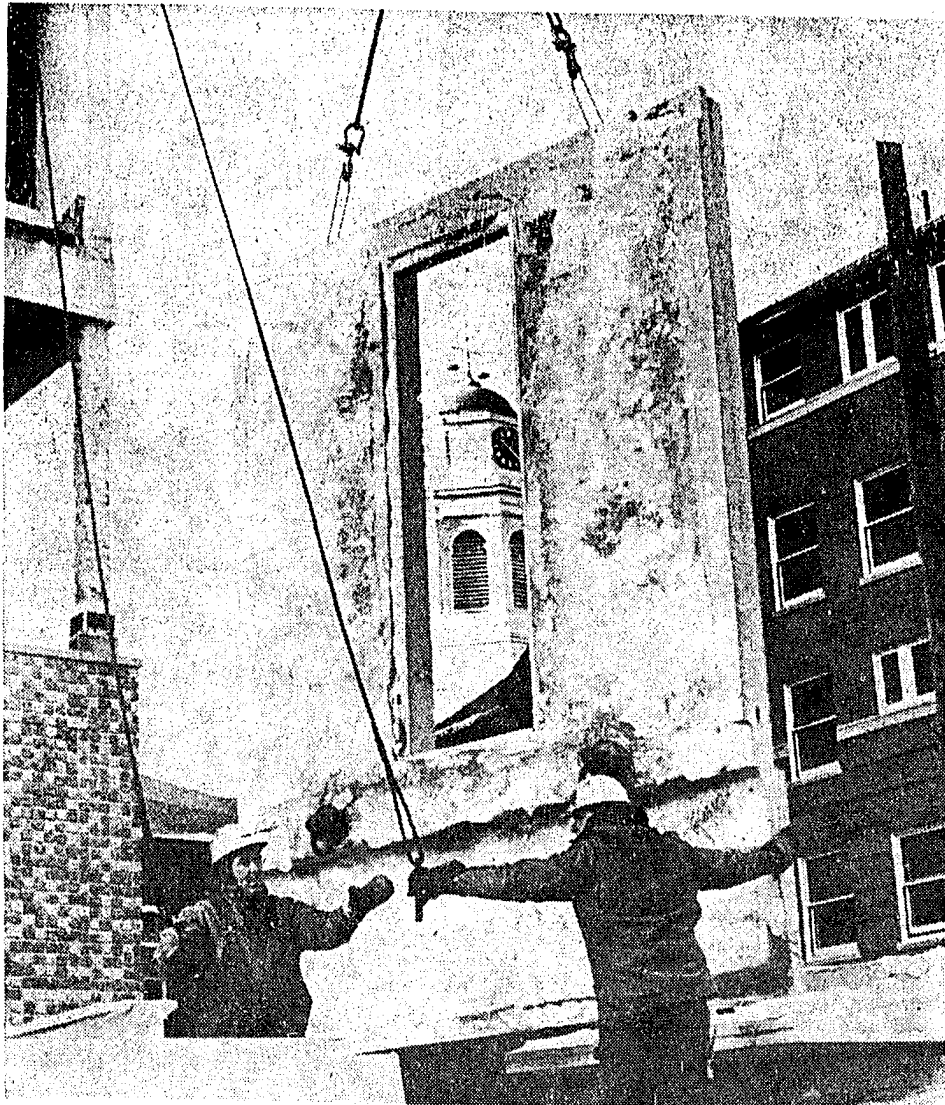
COURTHOUSE CONSTRUCTION — Workers prepare window panel before it's hoisted into place on upper story of new Middlesex County
